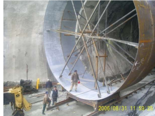
MOVING PENSTOCK D 9m into TUNNEL
