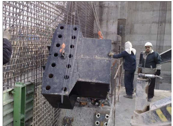
TRUNION BEAM INSTALLATION
