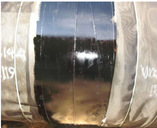
PAINTING on WELDED JOINT
