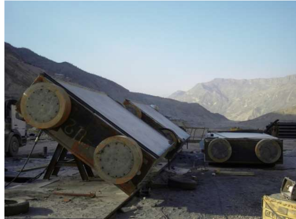
EMERGENCY GATE MONTAGE
