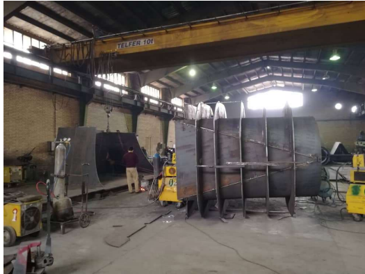
BOTTOM OUTLET TRANSITION
