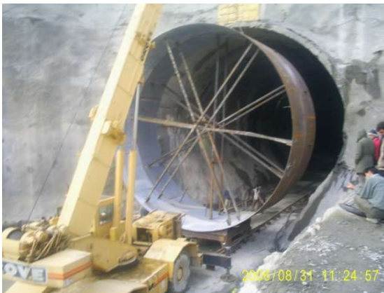
MOVING PENSTOCK D 9m into TUNNEL
