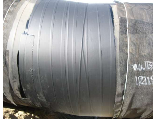
RAPPING on WELDED JOINT
