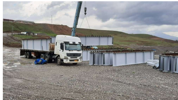
INTAKE TOWER BRIDGE
