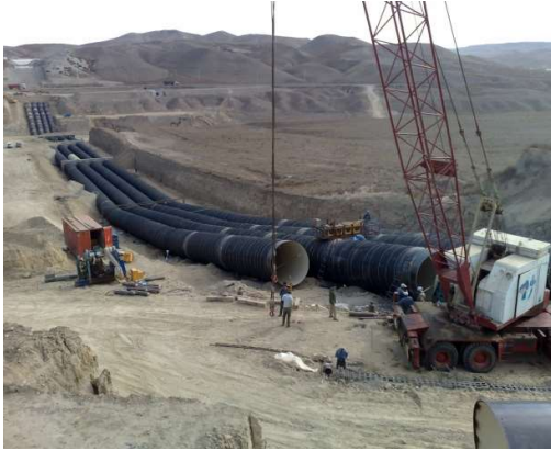
INSTALLATION OF PIPES
