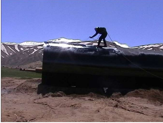
PAINTING OF PENSTOCKS
