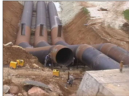
INSTALLATION OF PENSTOCKS
