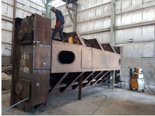
Khersan Dam Diversion Lower Part
