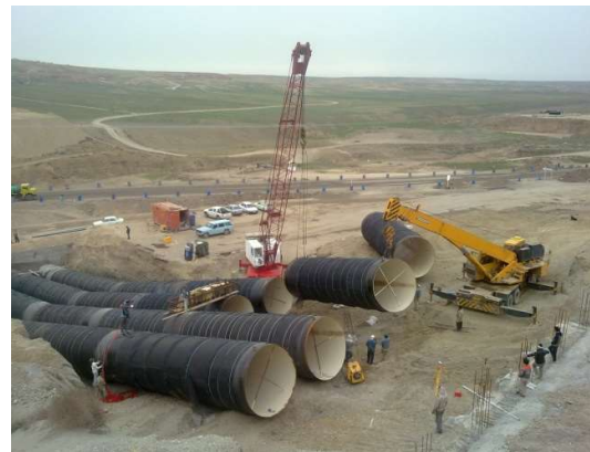
INSTALLATION OF PIPES
