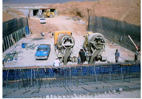
INSTALLATION OF PENSTOCKS
