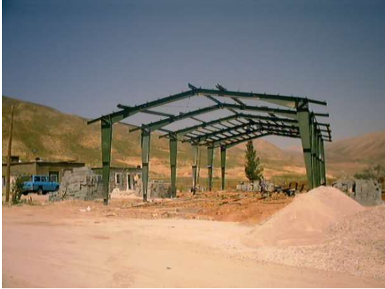
KOOHRANG STEEL STRUCTURE
