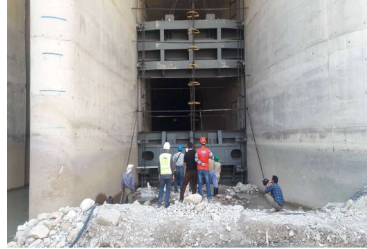
Khersan Dam Diversion Installation
