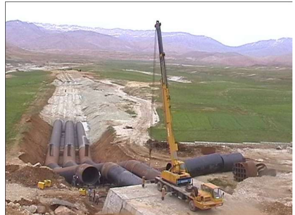
INSTALLATION OF PENSTOCKS
