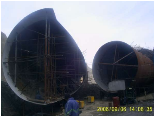
INSTALLATION OF Y - BRANCH
