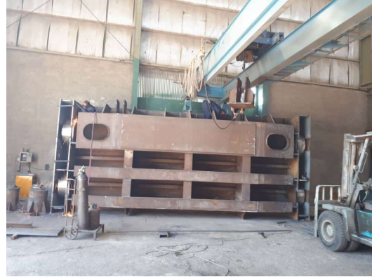
Khersan Dam Diversion Upper Part
