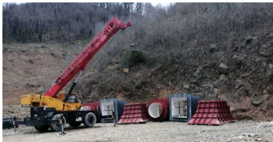
BOTTOM OUTLET TRANSITION
