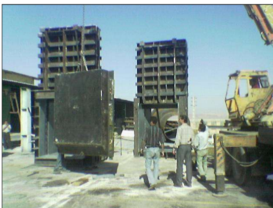
DRY TEST OF GATE & CASING
