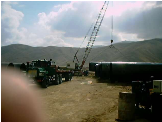
INSTALLATION OF PENSTOCKS
