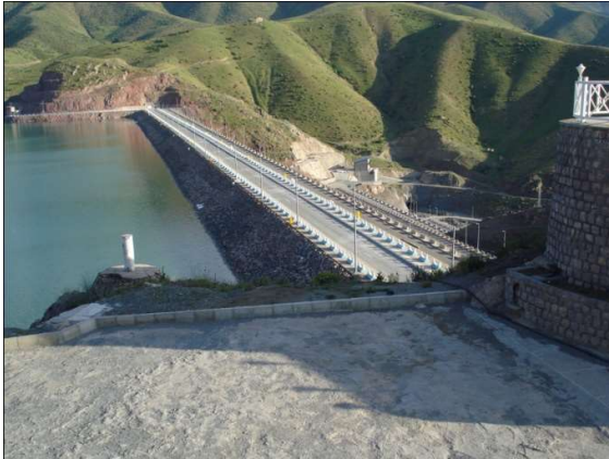
DAM UPSTREAM VIEW
