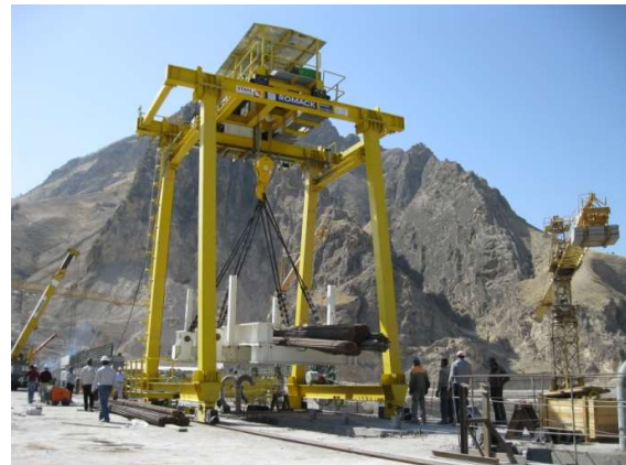
GANTRY CRANE INSTALLATION
