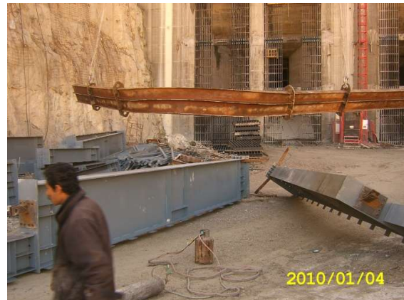
ARMAND BRIDGE BREAK DOWN
