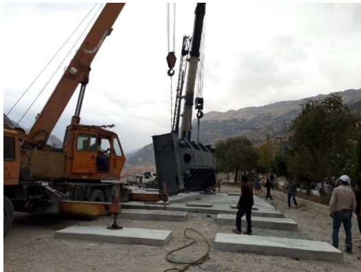
Khersan Dam Diversion Installation
