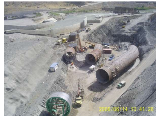
INSTALLATION OF PENSTOCKS
