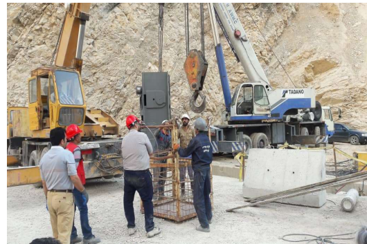
Khersan Dam Installation
