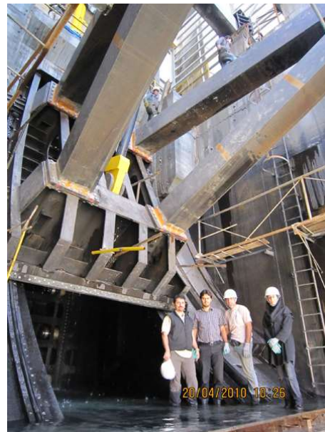
RADIAL GATE OUTLET
