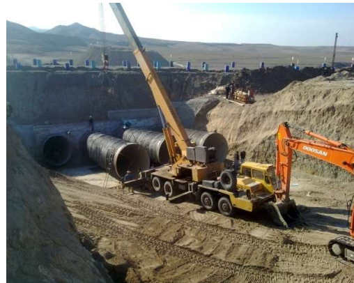
INSTALLATION OF PIPES
