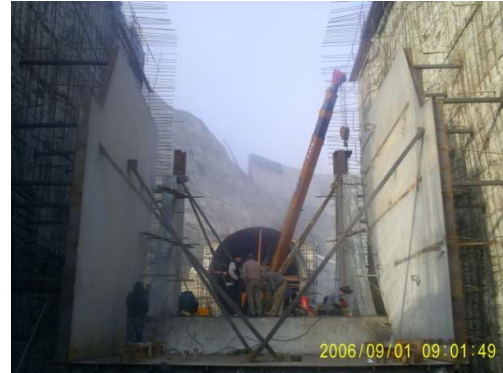
INSTALLATION of RADIAL GATE CASING
