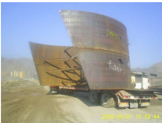
TRANSPORTATION OF PENSTOCKS
