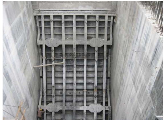
RADIAL GATE STRUCTURE
