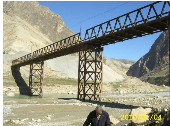
ARMAND BRIDGE BREAK DOWN
