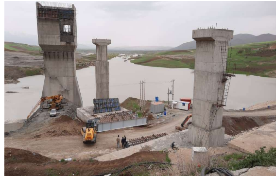
INTAKE TOWER BRIDGE
