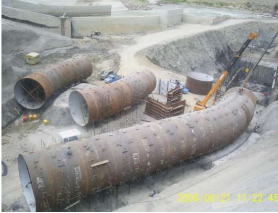
INSTALLATION OF PENSTOCKS
