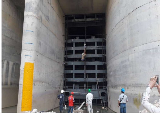
Khersan Dam Diversion Installation
