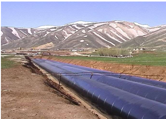
INSTALLATION OF PENSTOCKS
